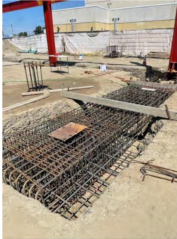
Classrooms Building Footing
