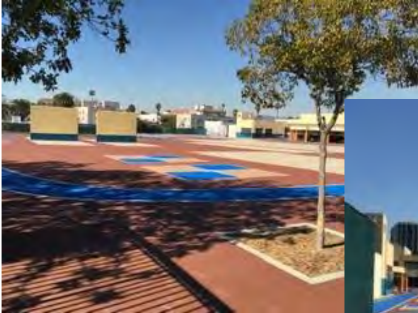
Southwest View of New Playground
