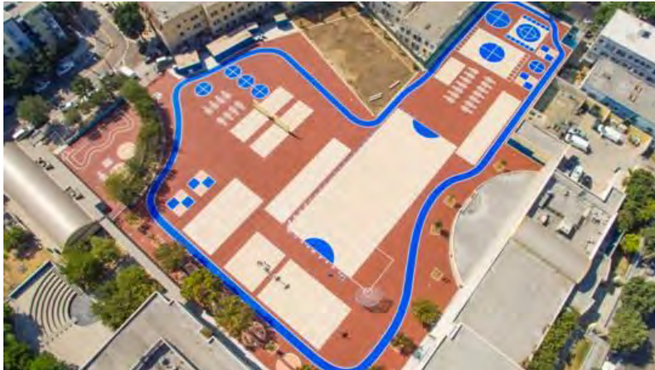
Aerial View of the completed playground with cool coating
