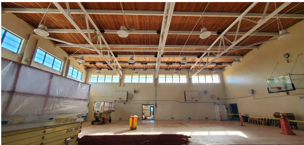
In Construction: Gymnasium Retrofit
