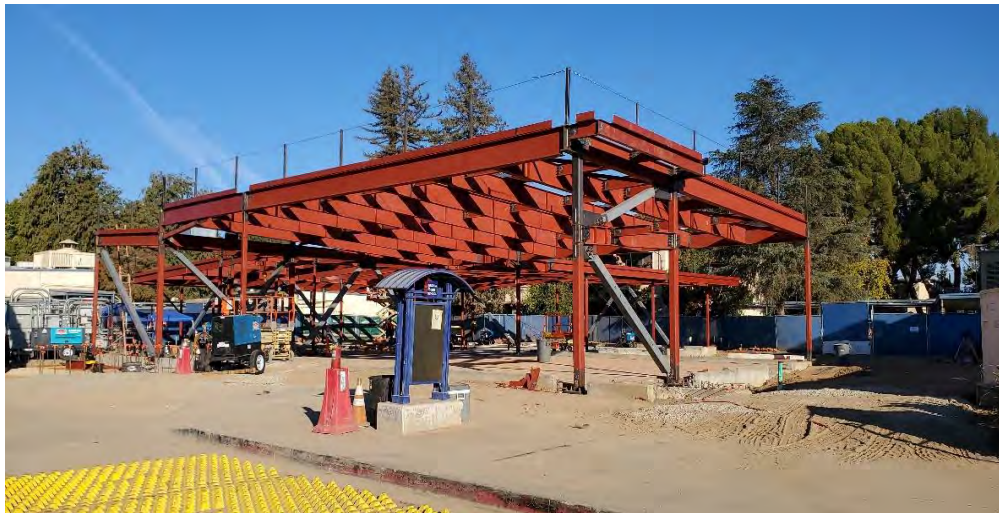
In Construction: New Cafeteria Steel Frame
