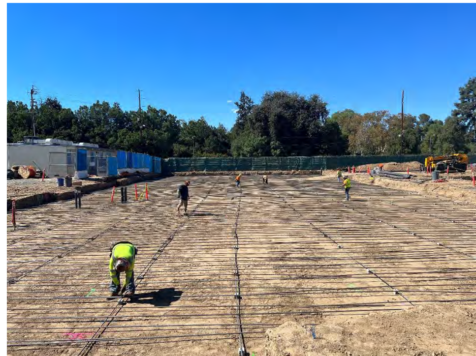
In Construction: New Classroom Building Foundation
