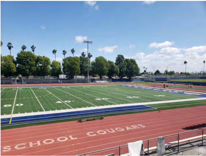
Synthetic Turf Field Replacement - South 50
