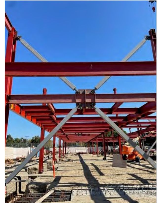
Classrooms Building Brace Frame
