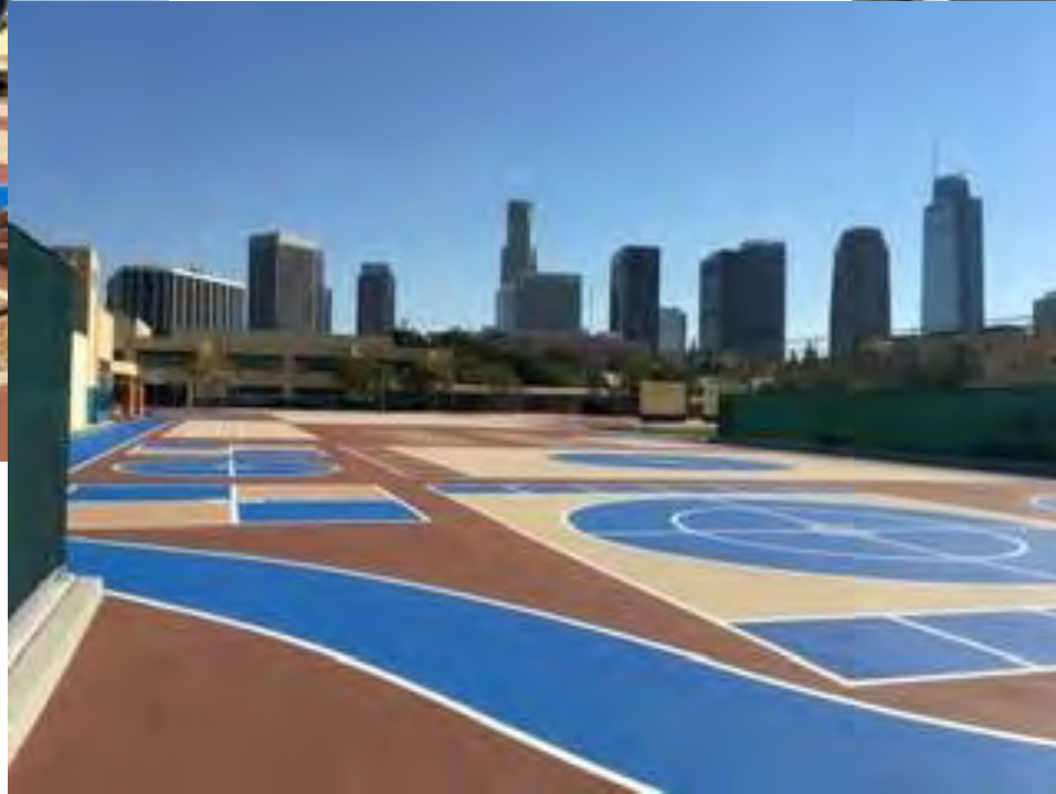
North View of Playground with Cool Coating Graphics
