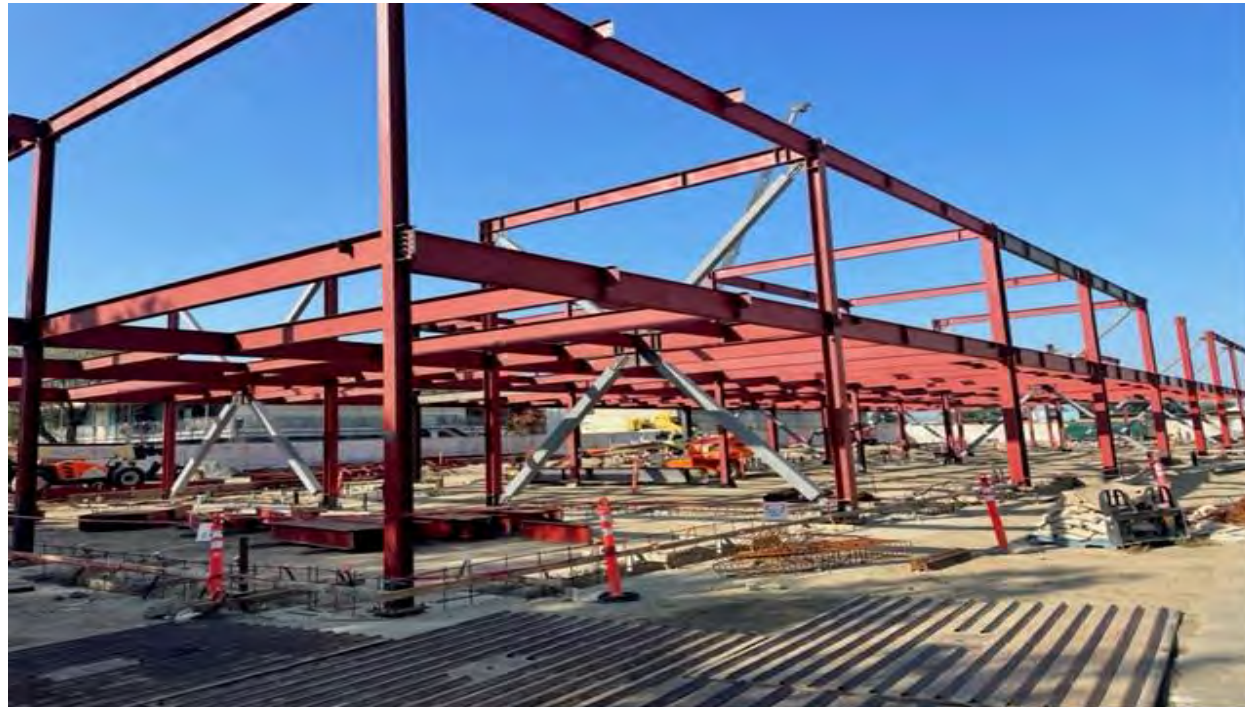
Two-story 21 Classrooms Building Structural Frame
